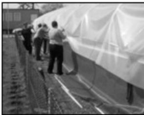
The polytunnel near completion
